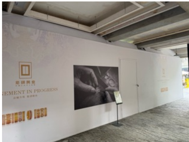
Figure 4: Laopu's new boutique in Xintiandi, Shanghai - under construction
