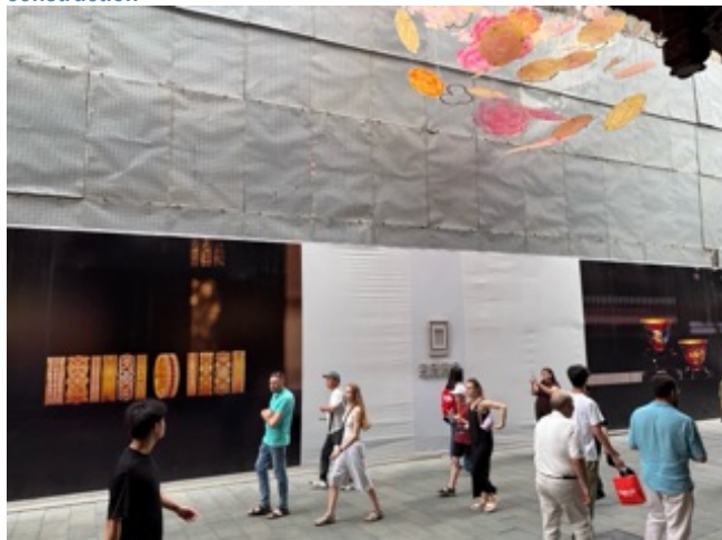
Figure 5: Laopu's new boutique in Yu Garden, Shanghai - under construction
